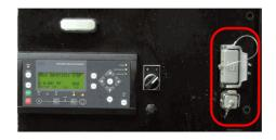
**NOTE** If the two sockets are mounted behind a door or hatch, make sure that enough space is available to close the door or hatch when the RMB cables are connected.
